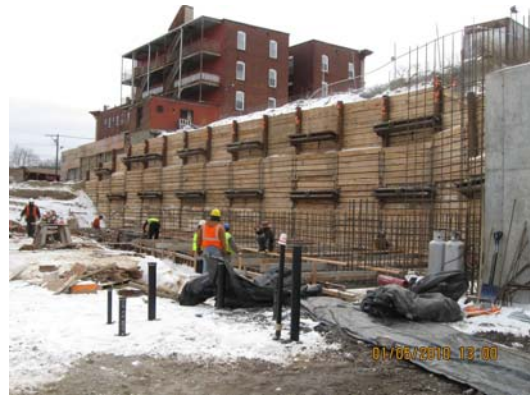
DUGGAN SCHOOL - L Line Footing Progress
