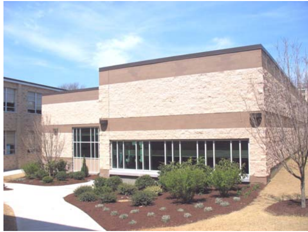
Left— Kennedy High School—as seen before the construction project began.
